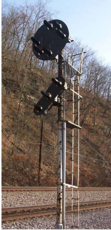
Figure 13. Color position signal with “yellow only” lower head
