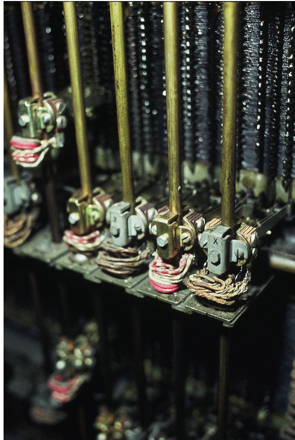
Figure 6. Selector brush assemblies
