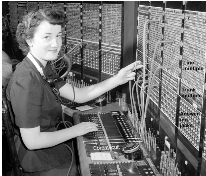
Figure 24. Manual switchboard, Vancouver, B.C., Canada (ca. 1947)
