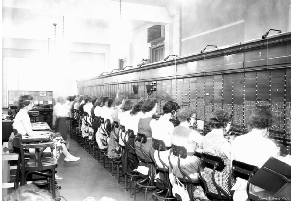
Figure 2. No. 1 common battery “A” switchboard
