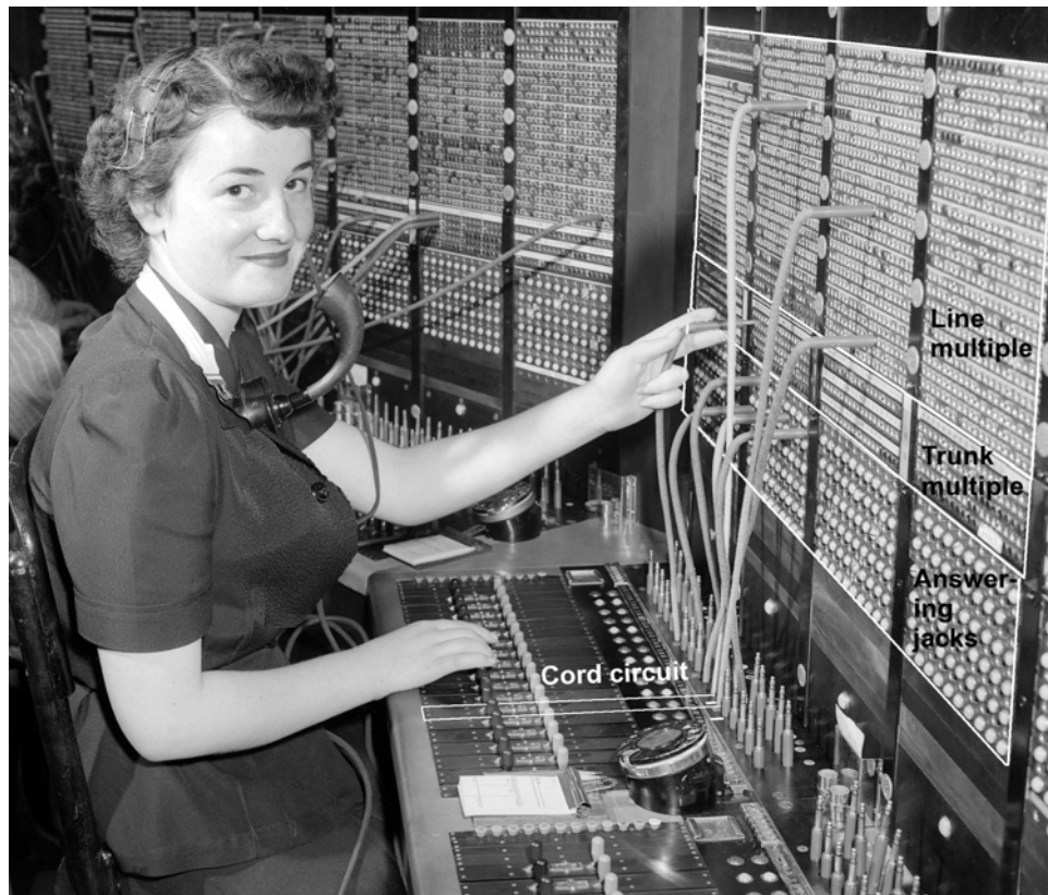
Figure 4. Automatic Electric common-battery switchboard (ca. 1947)
