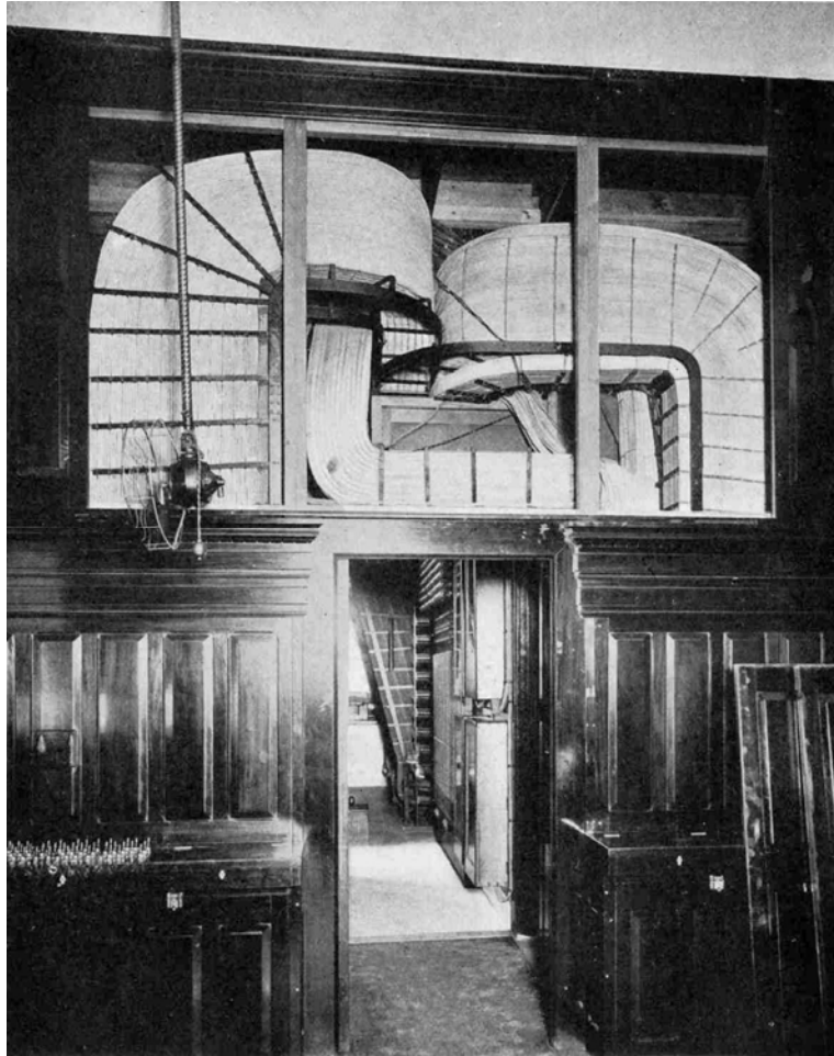
Figure 26. B and A switchboard multiple cabling
