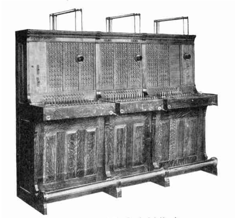
Figure 7. Three-position switchboard with suspended transmitters
