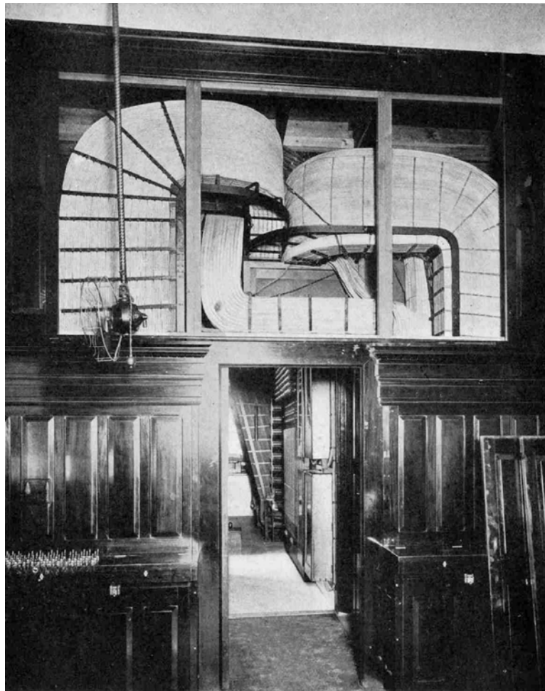
Figure 28. B and A switchboard multiple cabling
