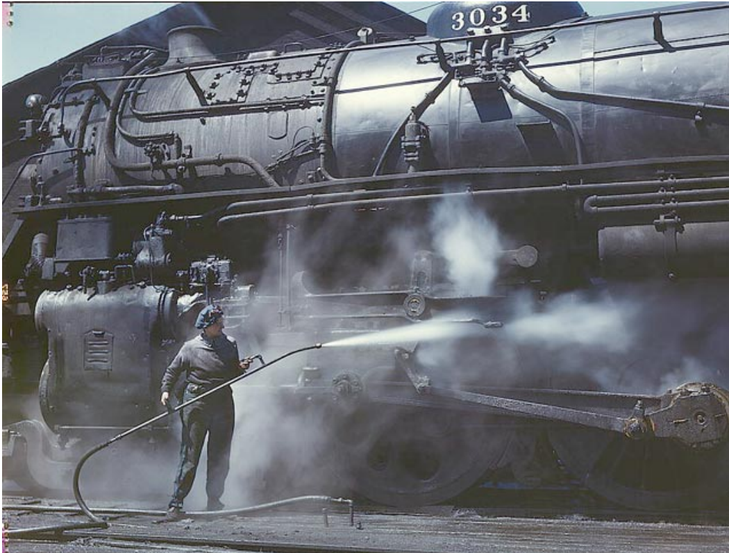
Figure 15. Steam cleaning a CNW class "H" locomotive
